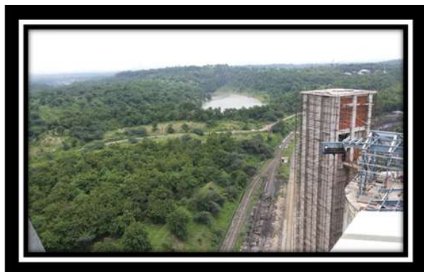
Bird's eye view of Plantation at Bharatpur & Balanda OCPs
